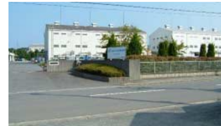
Production Plant No. 1 (left) & No. 2 (right)
