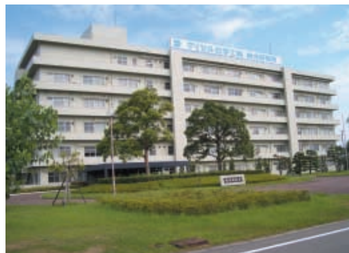
Daicel Chemical's Himeji Research Center is developing the aerobic oxidation technology utilizing NHPI catalyst.
